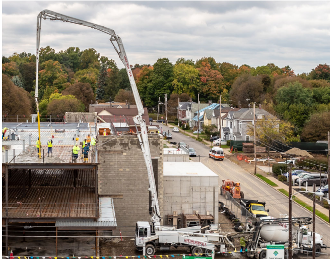
Our 36-Meter Truck Mounted Concrete Boom Pump
